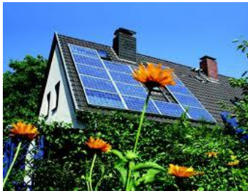
Panels parallel with plane of roof- Exempt
