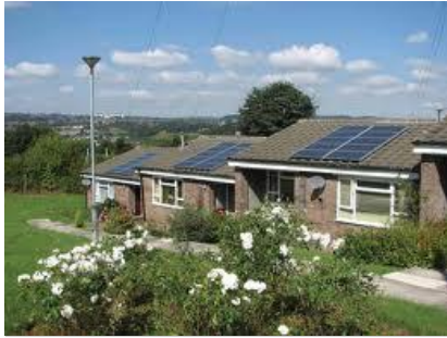
Different roof planes and independent roof structures.
