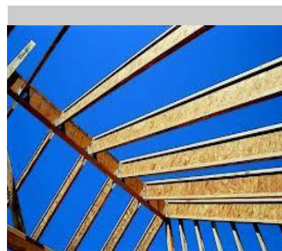
Different planes. Not independent roof structures.
